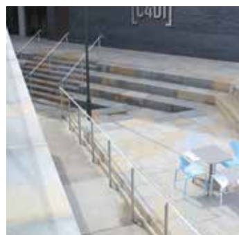
Centre for Digital Innovation, Government funded initiative (Bespoke cut sandstone paving, coping and steps)
