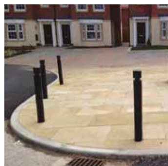
Miller Homes, Birkacre Park, Urban residential project (Bespoke cut paving and kerbs)
