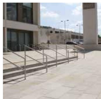
District Police Headquarters (Bespoke cut paving, tactile paving and steps with granite inserts)
